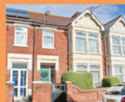
£240,000 Kenyon Road Three-bedroom house
